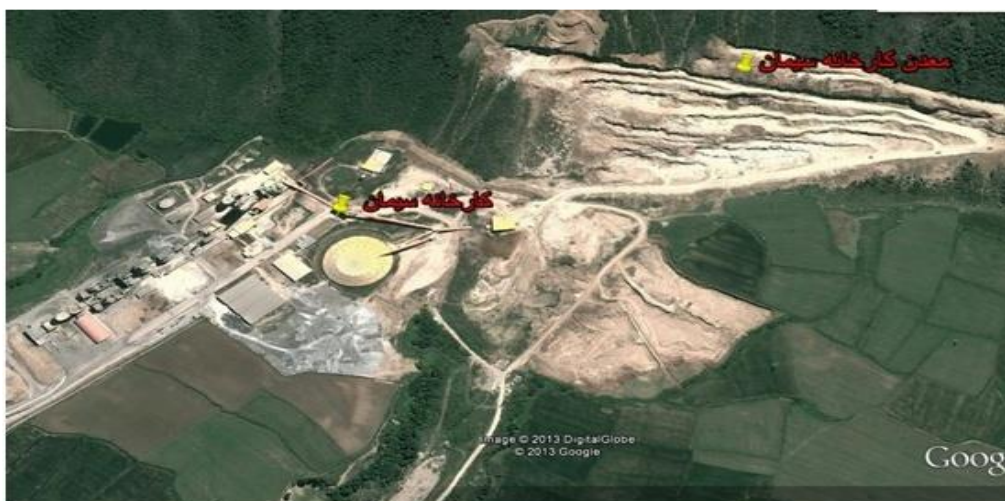
Fig. 2: Cement and mine extraction raw materials
