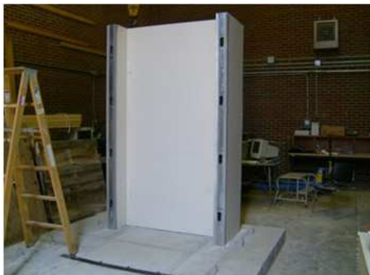
Fig. 3. Constructed partition wall
