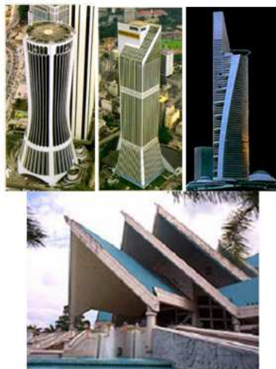
Fig. 18. Tabung Haji, Maybank, Menara Telekom and Balai Seni Lukis
