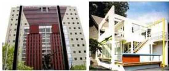
Fig. 11. Portland Building, Benacerraf House-Michael Graves
