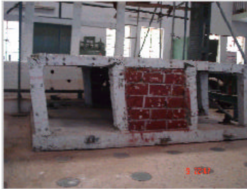
Fig. 10: Cracks and deflected shape of full frame
